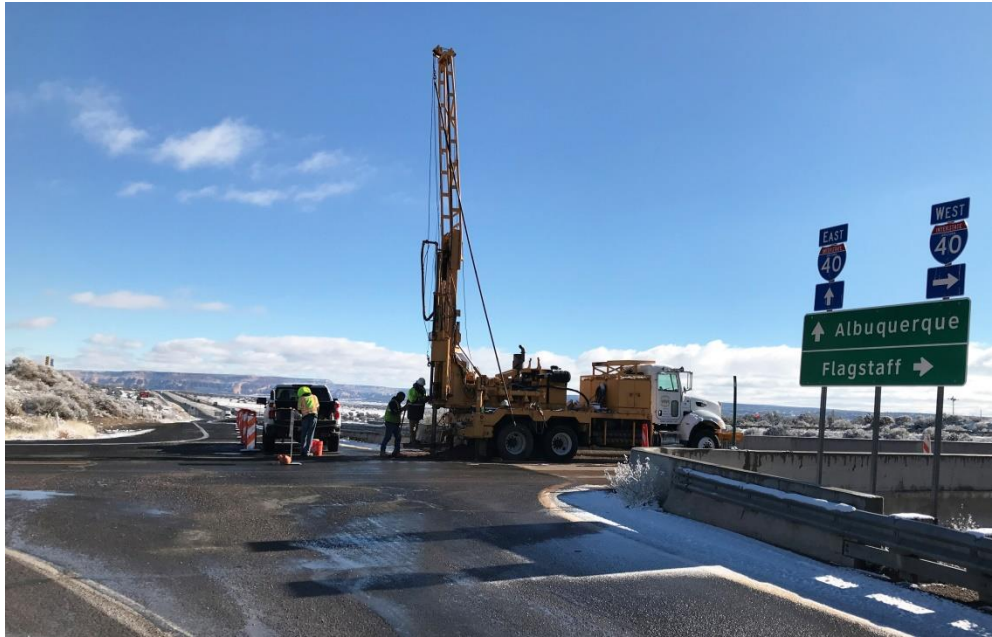
Figure 2: Drilling activities near the location of Abutment 1
