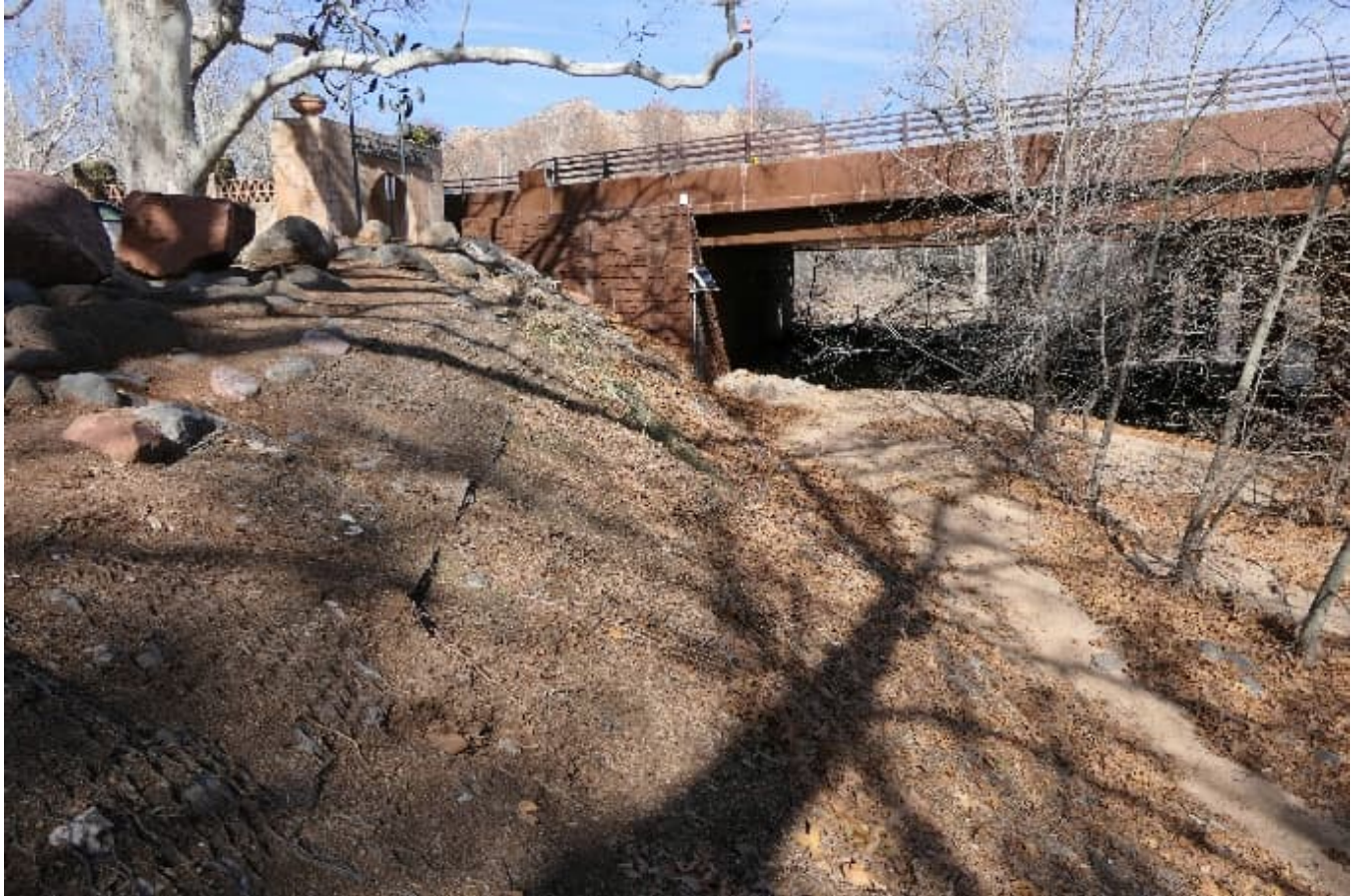
Figure 6: Parking lot fill looking north with gabion mattress
