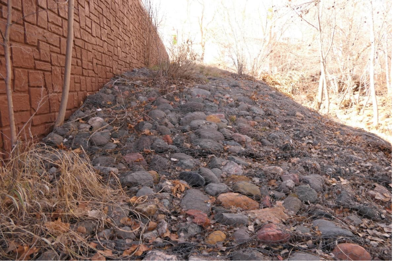
Figure 8: Access ramp and fill on north side of SR 179
