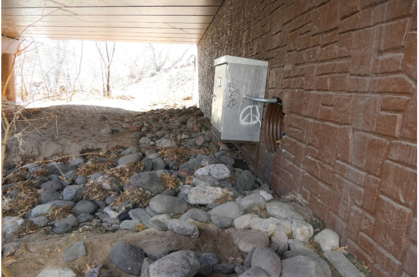
Figure 7: Coarse-grained rock in front of abutment wall
