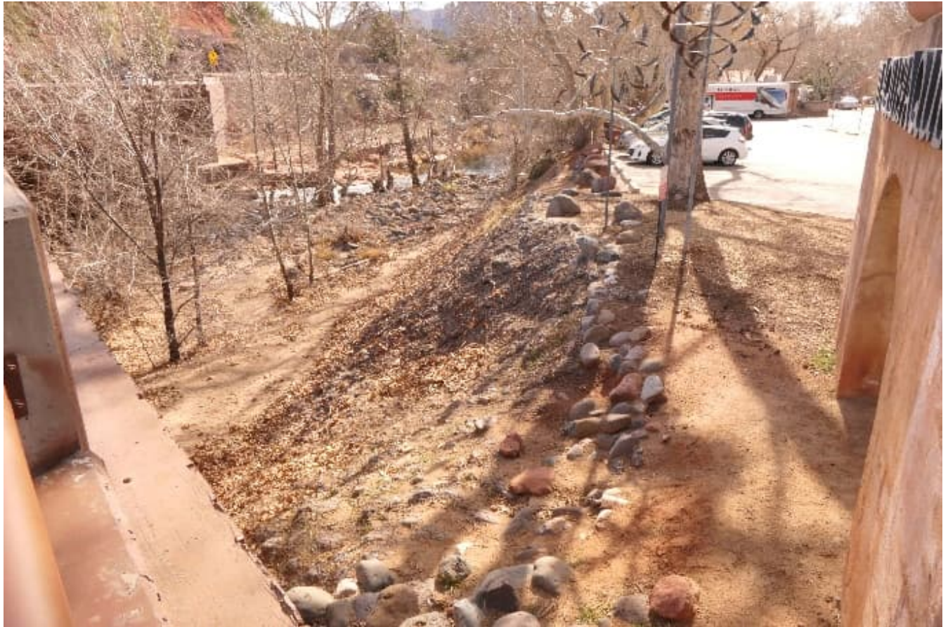
Figure 5: Parking lot fill looking south
