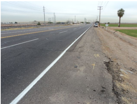
Picture 1 – Near 107th Ave.; Facing East
