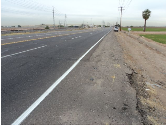
Picture 1 – Near 107th Ave.; Facing East
