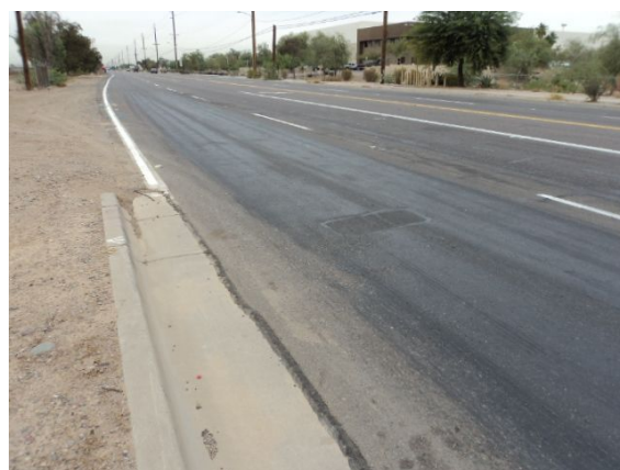
Picture 4 – Near 91st Ave.; Facing West
