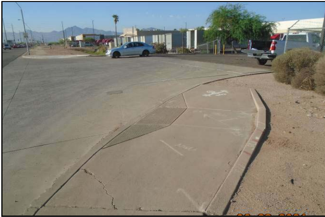
Picture 1 – 91 st Avenue, driveway near station 330+00, left of centerline.
