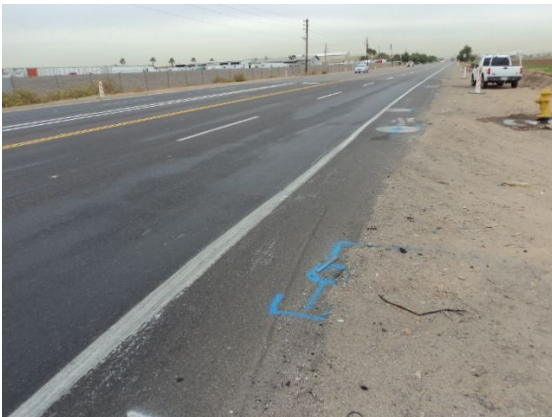
Picture 7 – Near 83rd Ave.; Facing East
