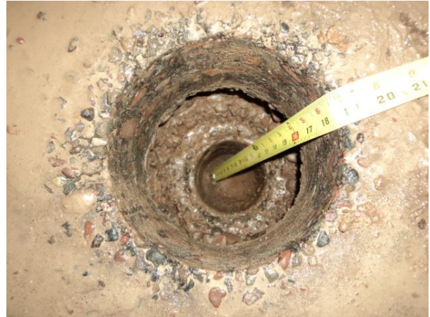
Picture 4 – Close-up of Picture 3
