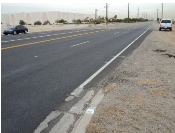
Picture 3 – Near 99th Ave.; Facing East
