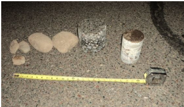
Picture 5 – AC and PCCP Cores Obtained at C9. Oversized rock (cobble) were encountered in the lower portion of the ABC. The top of the PCCP included a roughly ¼-inch thick layer of AC.
