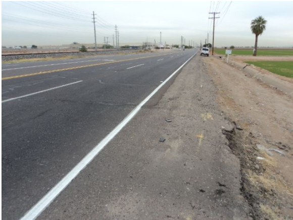
Picture 1 – Near 107th Ave.; Facing East
