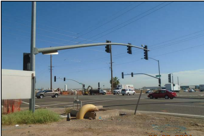
Picture 3 – Intersection of 91 st Avenue and MC85 / Buckeye Road.
